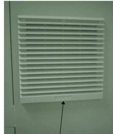
Unclip air filter
